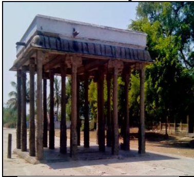
Figure 18: Sixteen Pillar Hall
