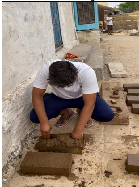
Figure 3: Transfer of the well-mixed material into brick molds
