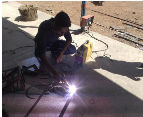
Figure 2: Arc Welding Working Process
