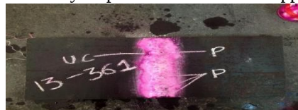
Figure 11: Inspection of weld for MS as filler rod
